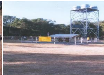
Water Storage Tower
